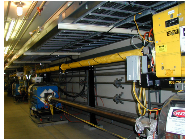
50 Gauss solenoid section
