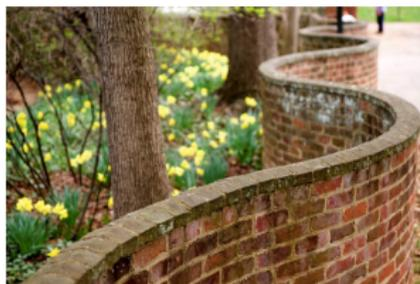
“These walls are called "serpentine" because they run a sinusoidal course, one that lends strength to the wall and allows [for it] to be only one brick thick, one of many innovations by which Jefferson attempted to combine aesthetics with utility.”
