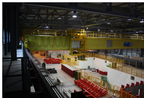
Construction of the extension of an existing building for office and laboratory
