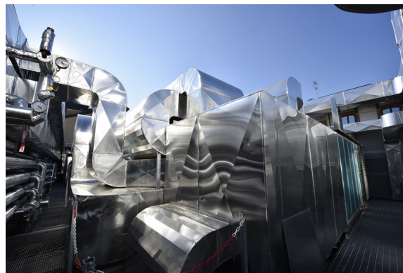
Construction of a new fitness center Virgin Active_ mechanical installations
