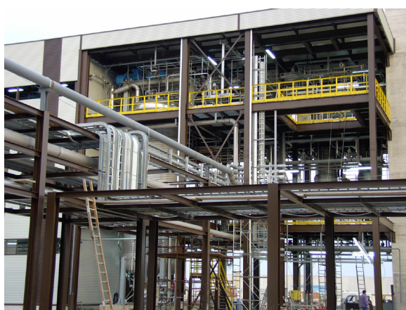
Installation of chemical plant
