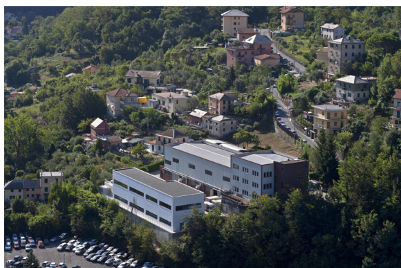
Columbus Superconductors headquarters in Genoa, Italy
