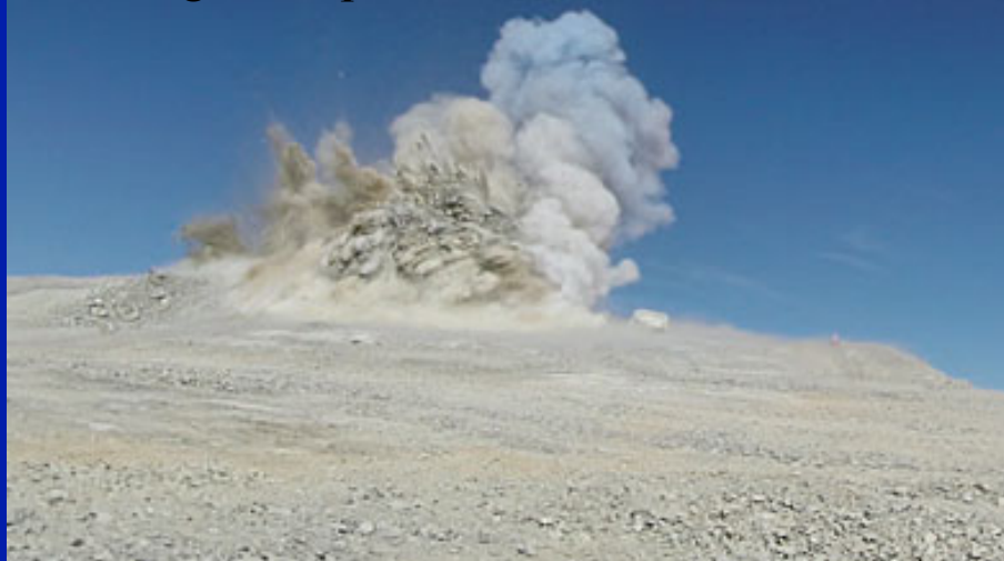
Blasting the top
