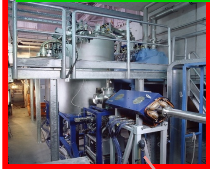
PIAVE Heavy Ion Injector
