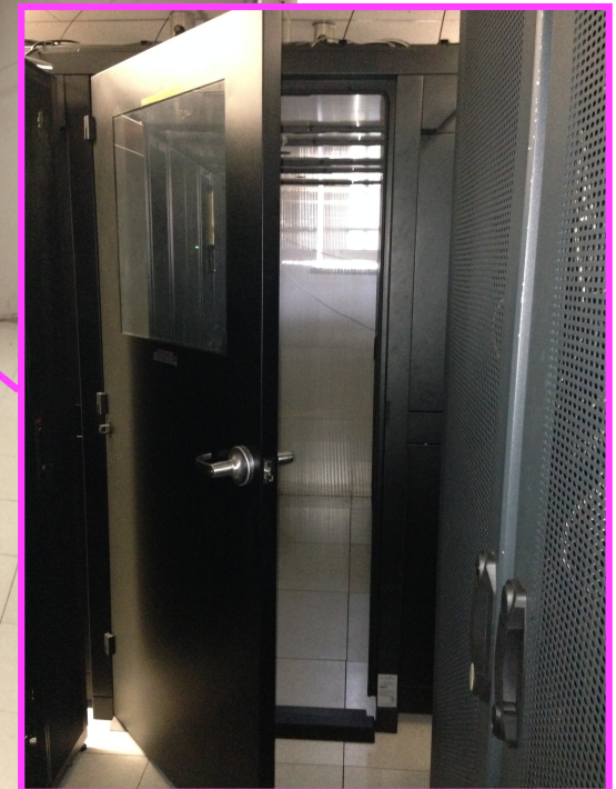
Water cooled hot aisle
