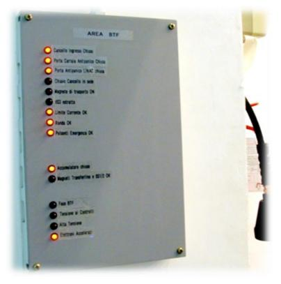
©Close the gate, turn the key clock-wise (once), and remove the key (you will need the other, smaller key, attached to it, for the next step)  Make sure that the "RONDA OK" led in the synoptic panel close to the gate is on, otherwise you have to repeat the search correctly
