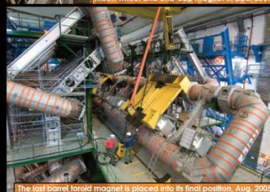
The last barrel toroid magnet is placed into its final position, Aug. 2005
