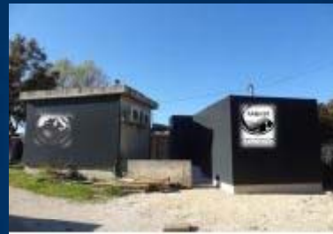
Power station of KM3NeT-Fr
