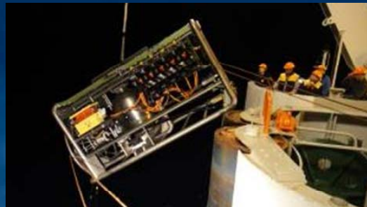
Deployment of node at KM3NeT-Fr
