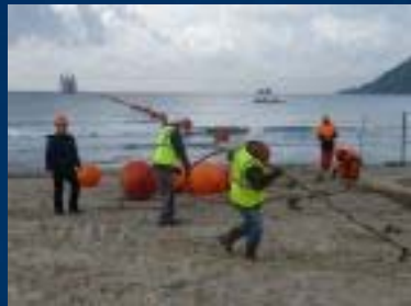
Deployment of the KM3NeT-Fr long-distance cable
