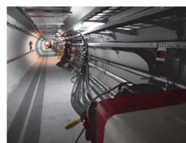
CNGS magnets dismantled, cables for AWAKE magnets installed (TT41)
