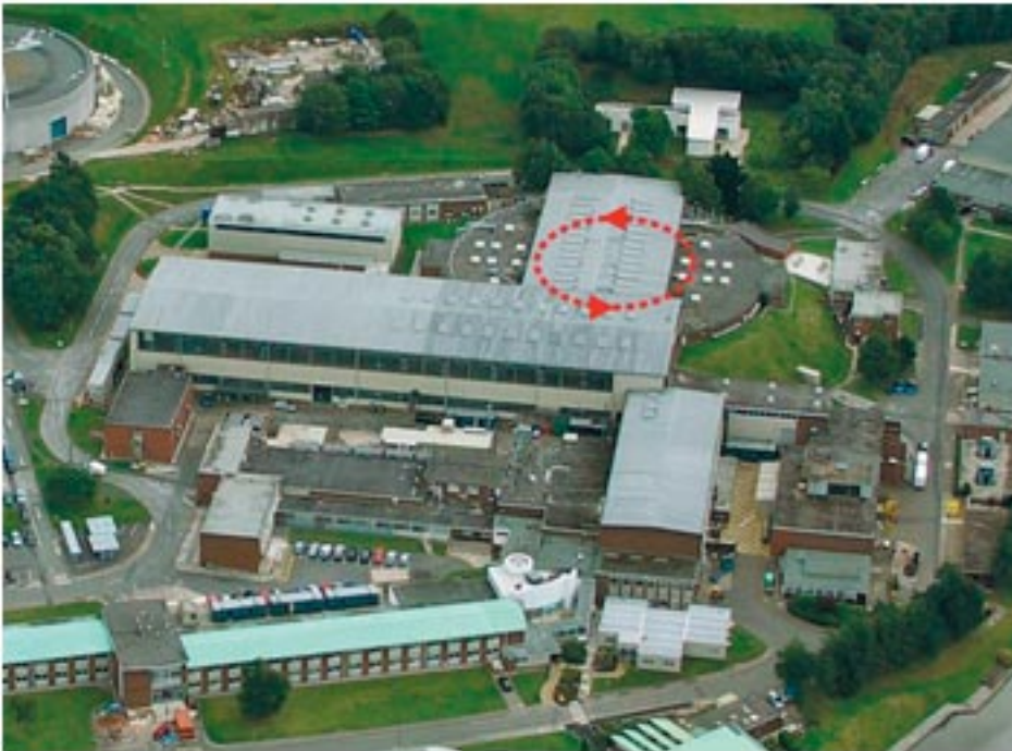
SRS storage ring at Daresbury (UK)
