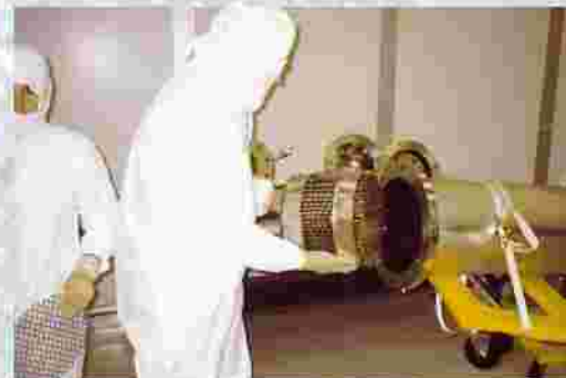
Assembly of distillation & water extraction columns in clean room
