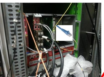
8 ethernet cables per board RJ45 terminated
