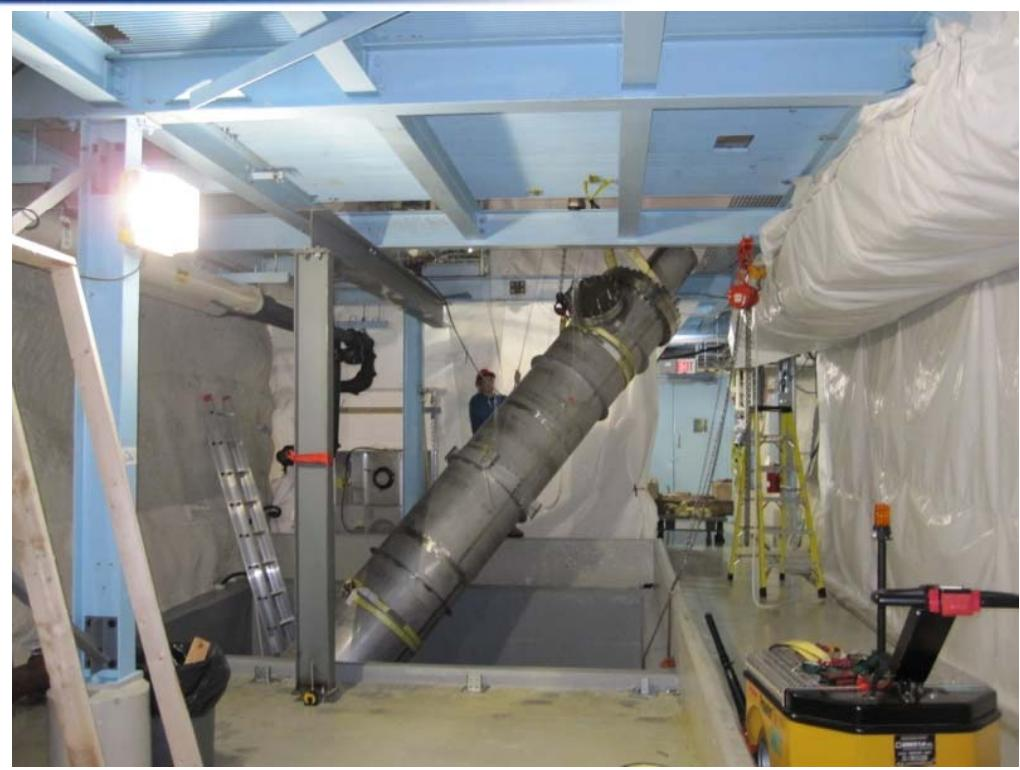
Development of a scaffold for cleaning internal surface of the acrylic vessel. AV now cleaned and ready for filling with water.
