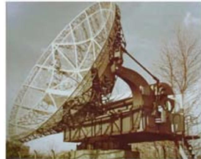
Wurzburg "Riese" Radar Antenna, 7.5 m diameter
