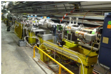
UA9 installation in the SPS
