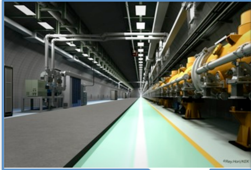
Acceleration units etc inside the 31 km tunnel
