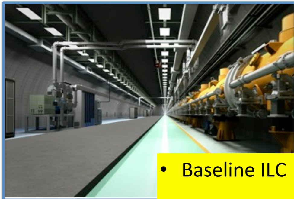
Acceleration units etc inside the 31 km tunnel
