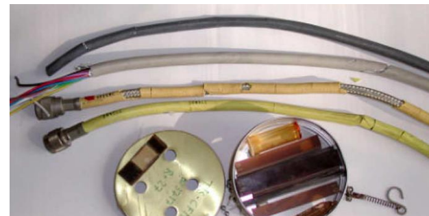
LEP damage to cables and magnet insulation ( NIM B )
