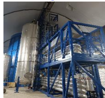
4) Gas stripping to remove Rn and O 2
