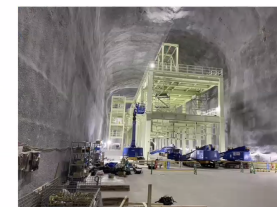
Water system installation
