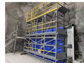
Test construction of the barrel lining
