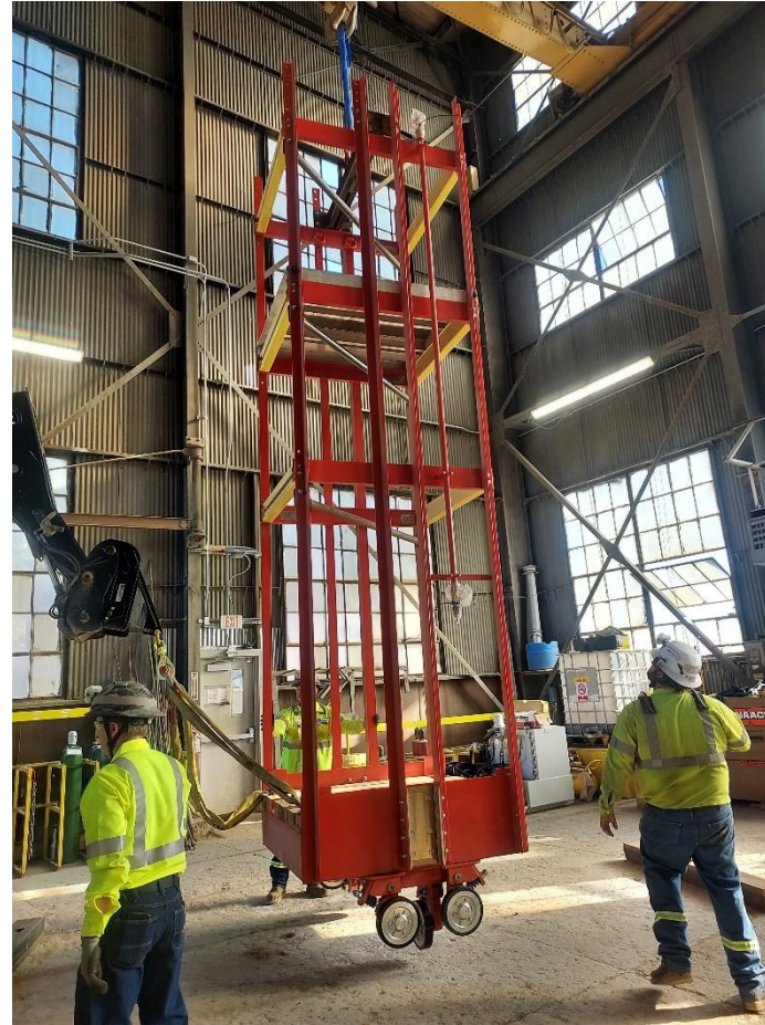
New Skip Cage Installation
