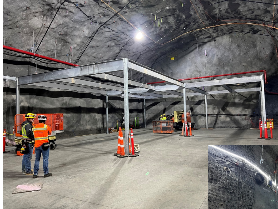
CUC Utility Building Steel Erection
