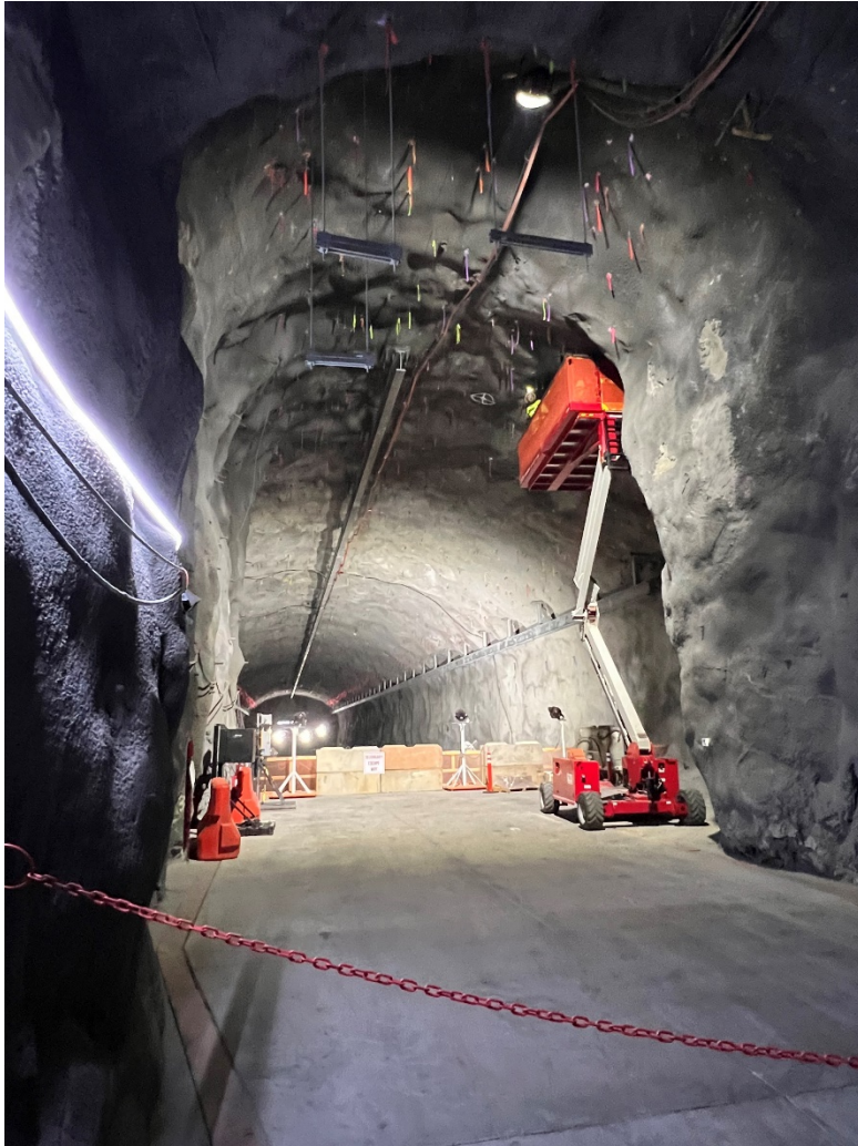
4850-14 Anchor Pull Testing
