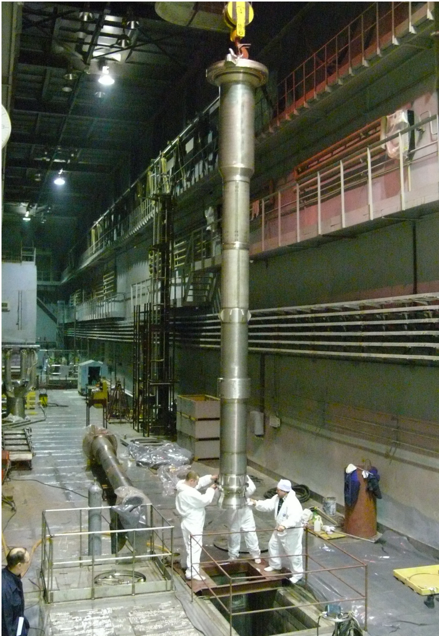
Technology hall. Mounting of the reactor body
