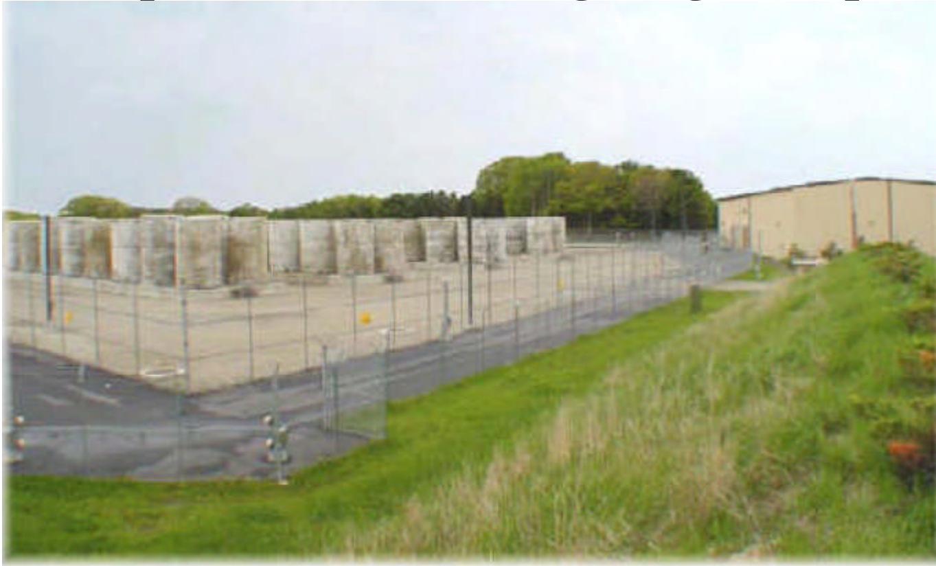
Figure 9. Dry cask storage of spent fuel. Two casks typically contain the equivalent of a year's spent fuel discharges from a 1000 MWe nuclear power plant. Comparison of the simplicity of interim spent fuel storage with the complexity of the huge reprocessing complex shown in Figure 6 makes it easier to understand the relatively low cost of interim storage. 87
