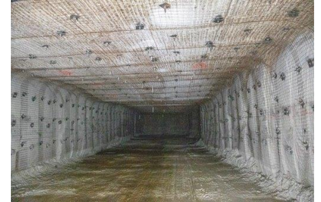
Stage 1 excavation – 8m wide by 5m high
