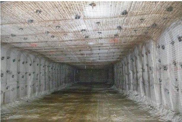
Stage 1 current status (as excavated)
