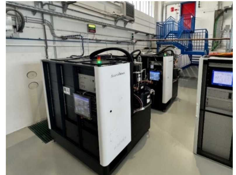
Installation at TEX
