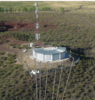
6 telescopes per building 4 buildings at edge of array (looking inward)
