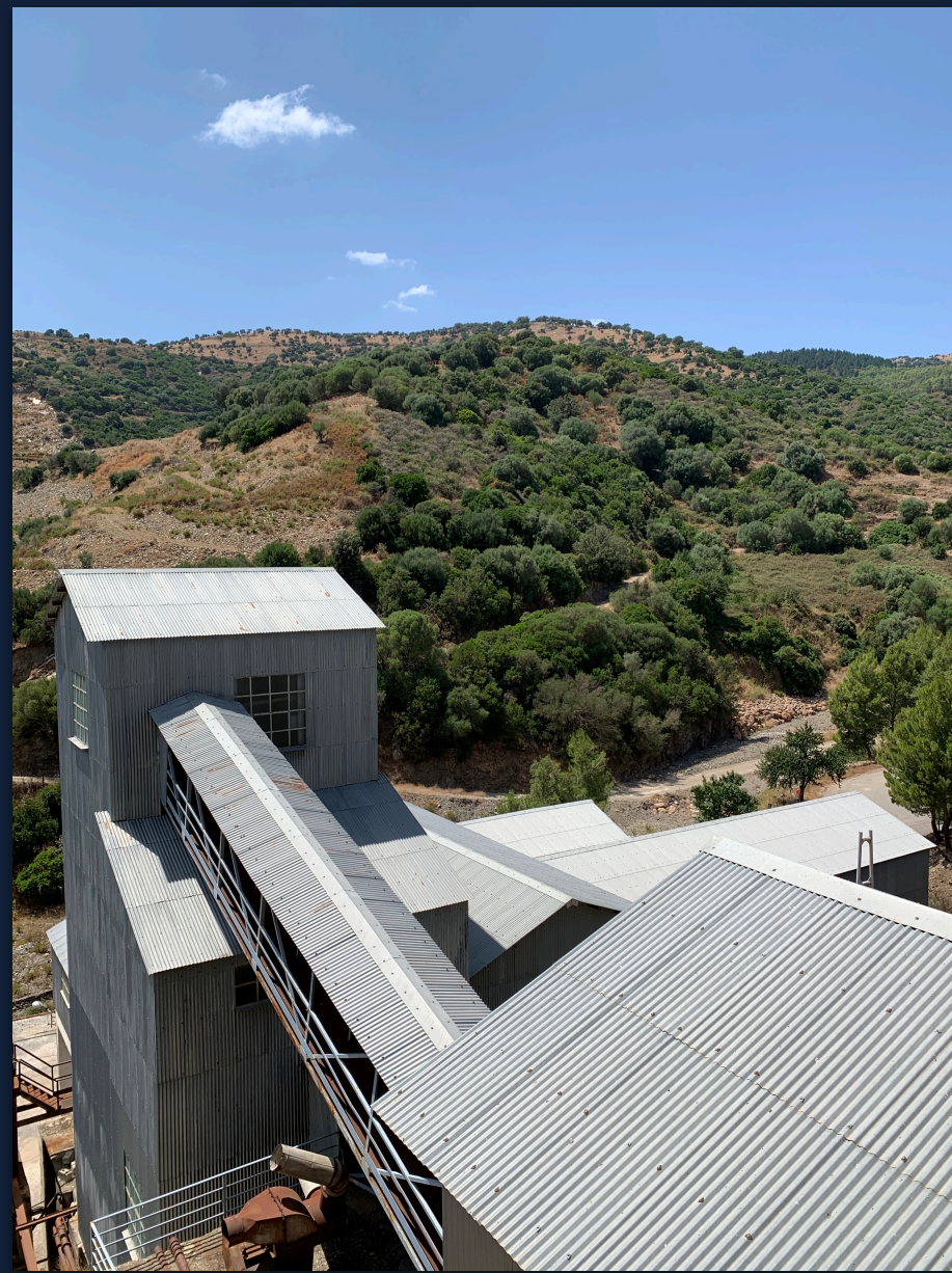
Former mineral processing unit
