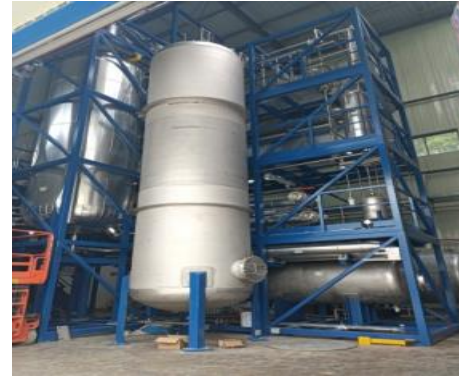
Distillation to remove radioactive impurities
