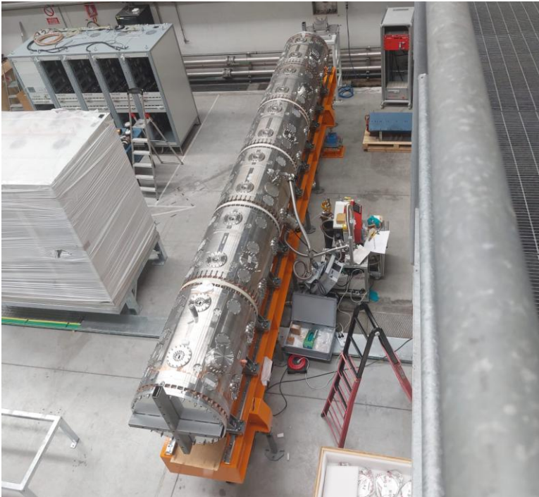
SPES RFQ installed at LNL (CW, 100kW, 80 MHz)
