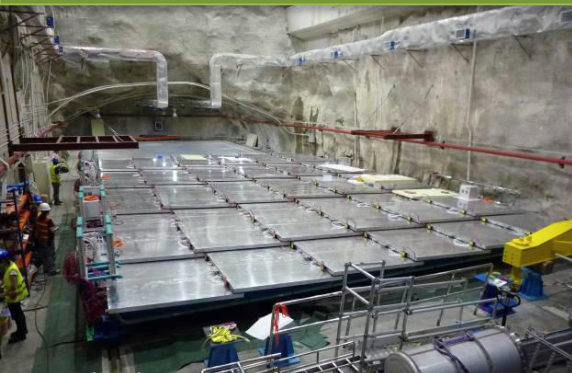
Covered with fully installed RPC detector
