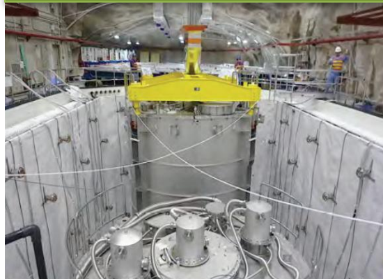
Filled AD installation
