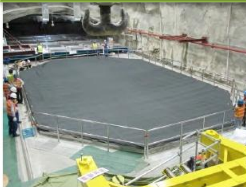
Pool cover installation
