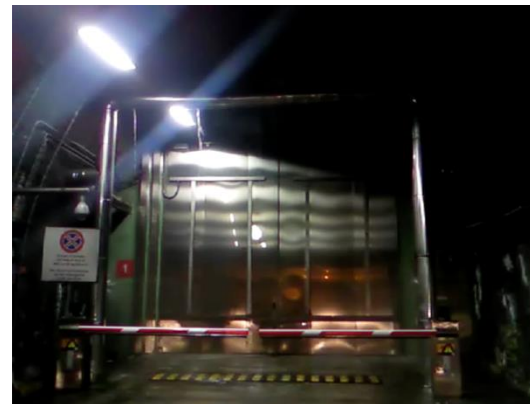
Niagara on the entrance/exit gates
