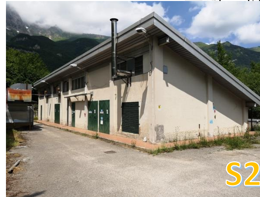
“Casale San Nicola” substation
