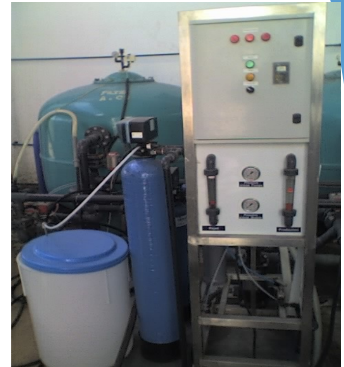
➤ Nanofiltration Unit (Filmtech NF40-40)
