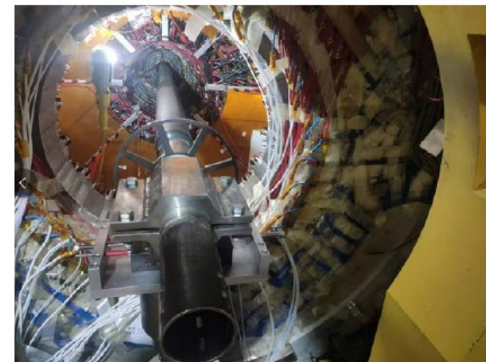
Install protecting sleeve for iMDC
