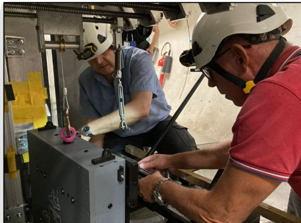
Emulsion target installation
