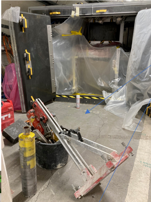
View of transported material to execute excavation works
