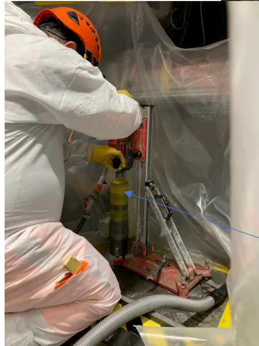
View of low-speed core drilling and direct dust removal
