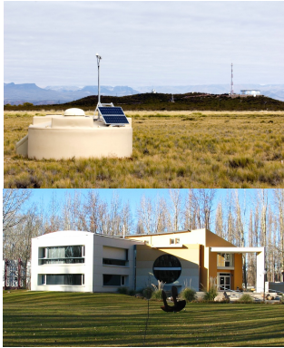
Control and Data Acquisition System (CDAS)
