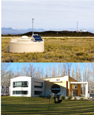
Control and Data Acquisition System (CDAS)
