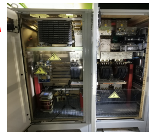
KLOE PS Dump resistor and contactors
