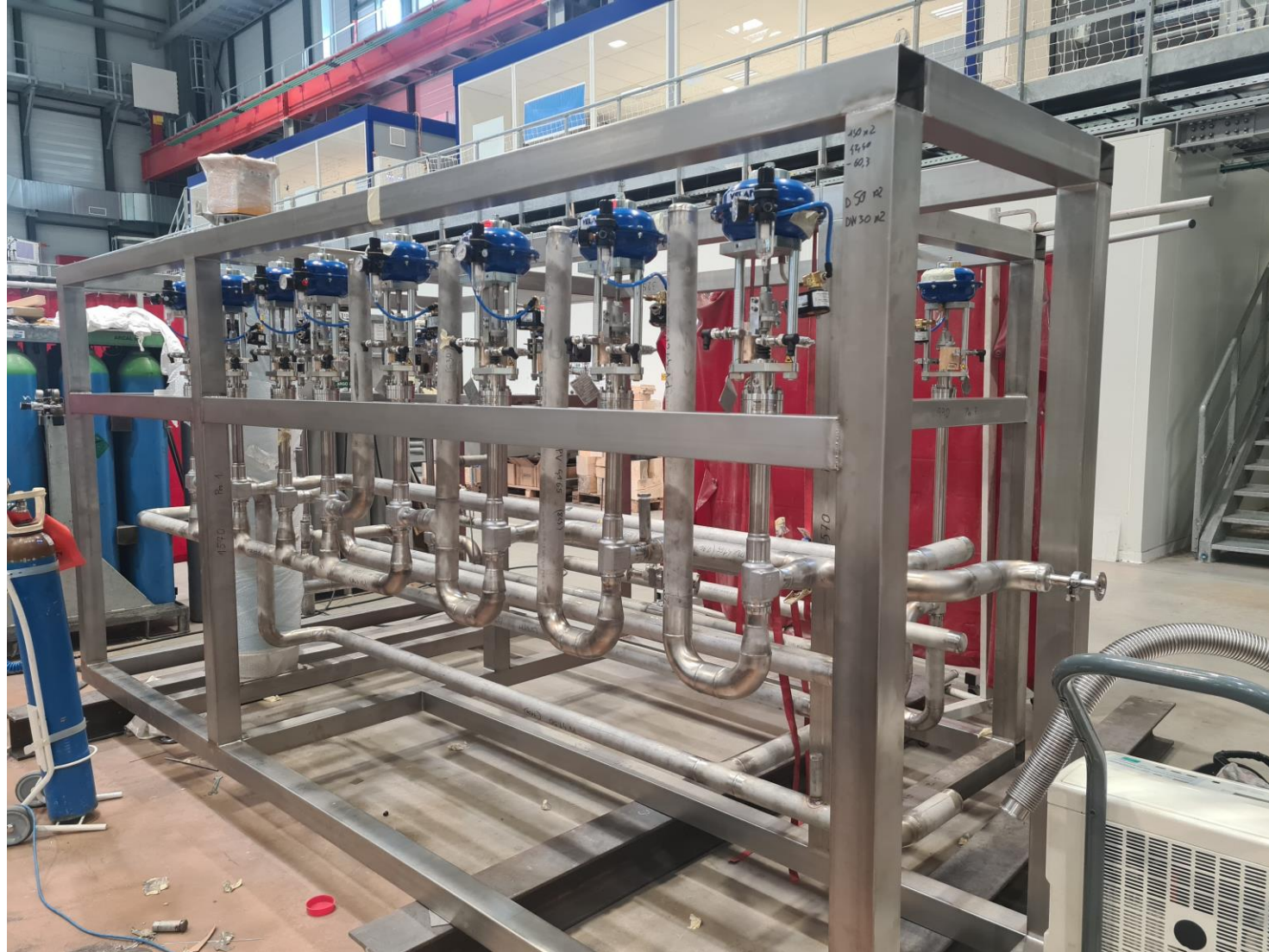
Fig. 2 – Warm panel, 1 st skid fully assembled, ready for testing.
