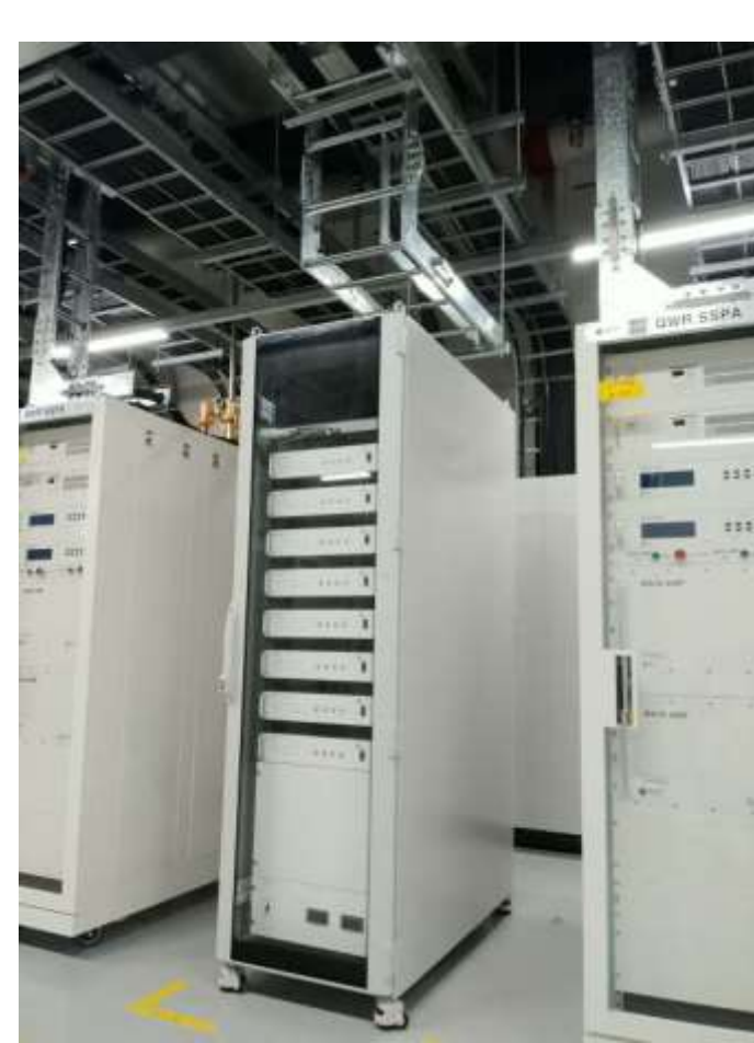
Installed LLRF
