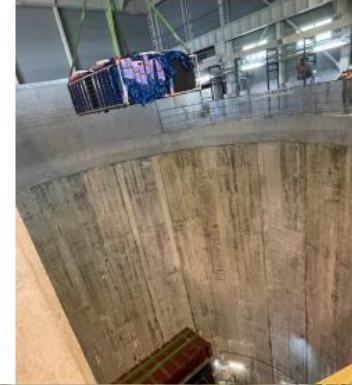
Super-FGD installation (October 2023)
