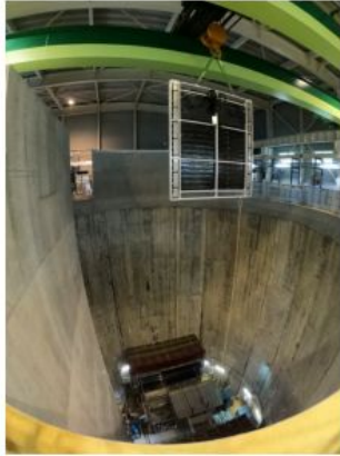
TOF installation (July 2023)
