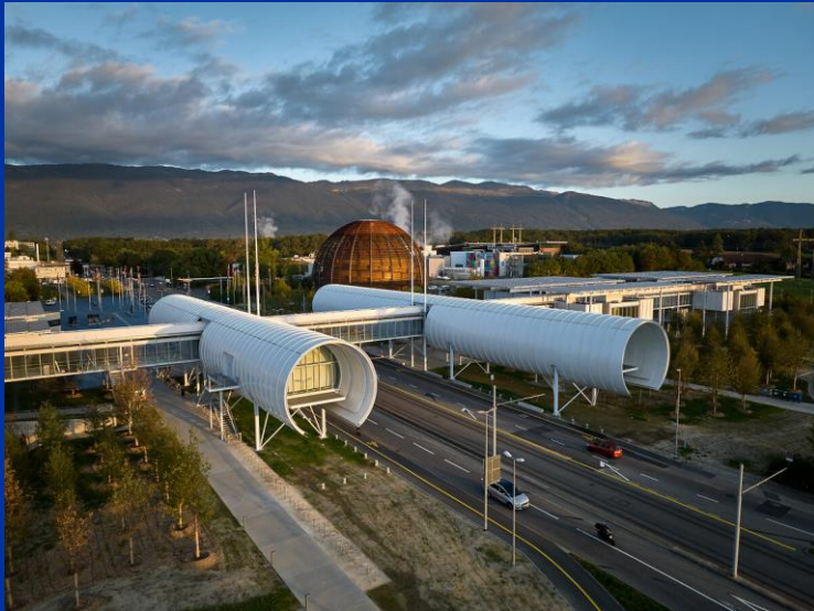
CERN Science Gateway designed by Renzo Piano Building Workshop
