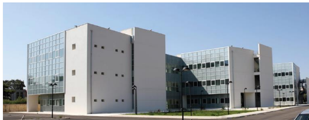
Clean Room Lab @ Dhitech (High-Tech District) □
