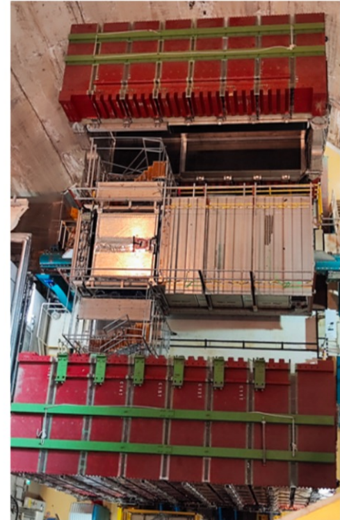
ND280 after lowering of top HATPC 2024.4.25
