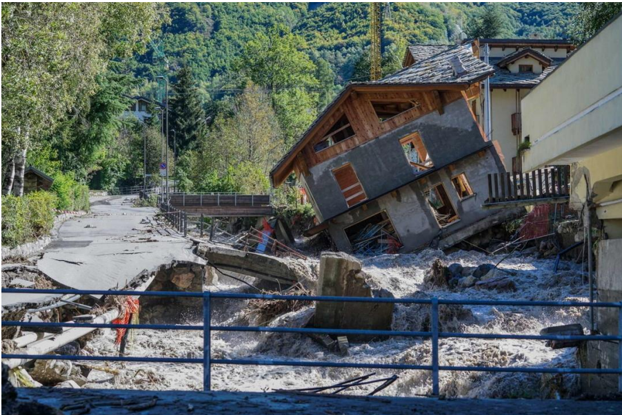
Flooding in Limone (CN) after the storm Alex, Oct 2020
