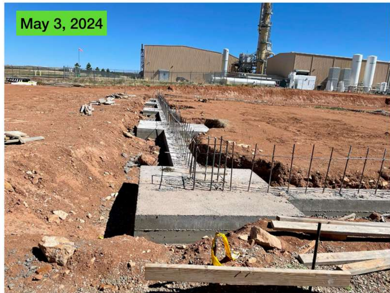
Concrete footings cast along gridline A
