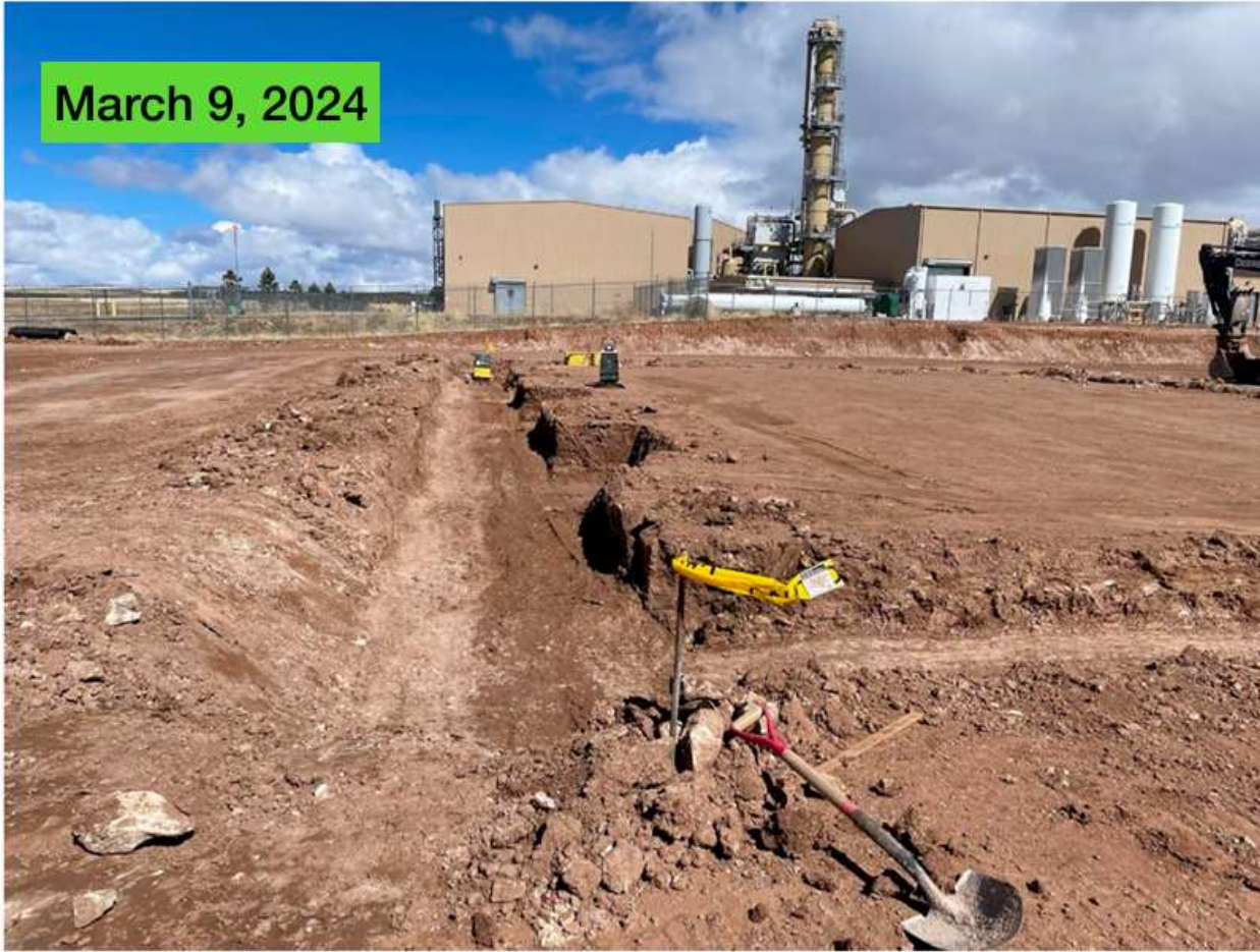
Footing excavation in progress
