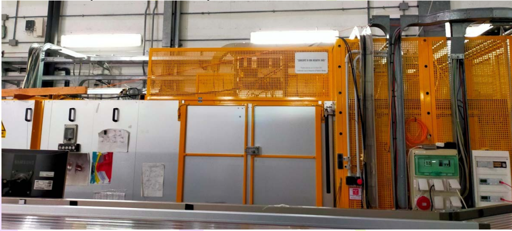
NIO1 external installation
