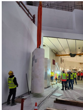
installation S-FRS lateral shielding blocks, May'24
