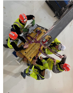
transport of the first quadrupole magnet in tunnel, Mar'24
