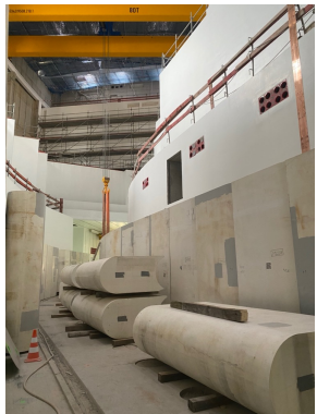
installation S-FRS lateral shielding blocks, May'24
