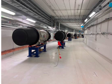
installation of SIS100 dipoles Apr'24
